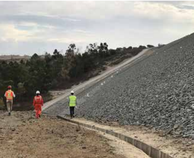
Neves-Corvo – Tailings Facility
