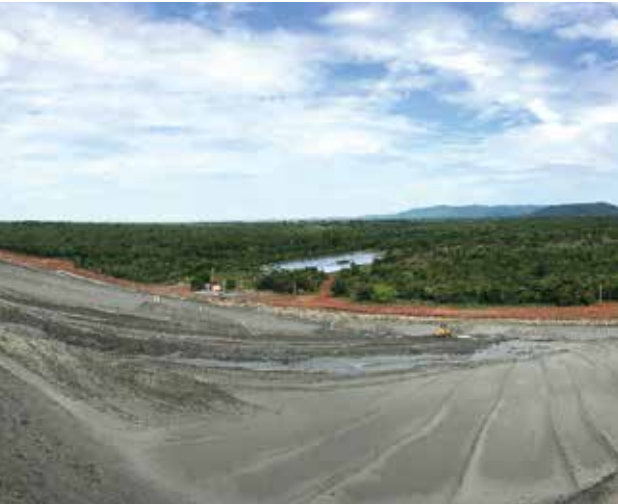
Chapada – Tailings Facility
