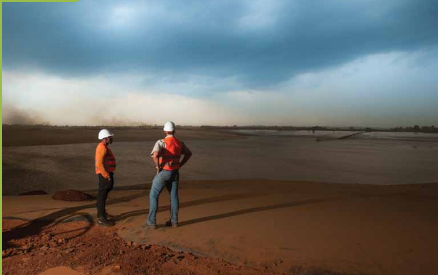
Tailings dam at Loulo, Mali.
