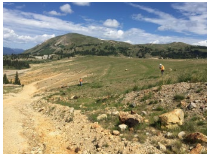
A company tailings engineer and a third-party inspector perform an annual tailings stewardship assessment at the Robinson impoundment at Climax, which has been inactive since the 1970s and was reclaimed in the 1990s.
